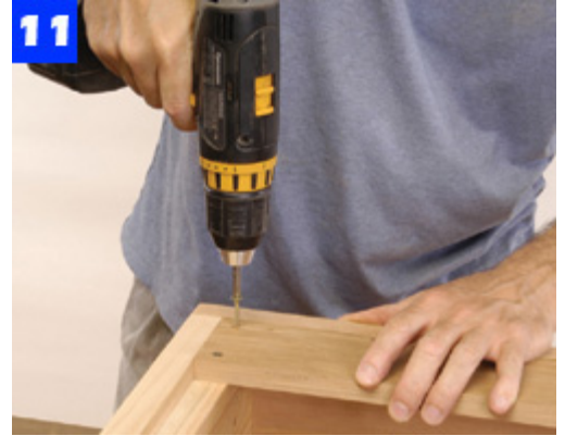
Screw the foot rails to the cleats. Note that the back edge of the rear chair foot rail is beveled to fit the back rail.
